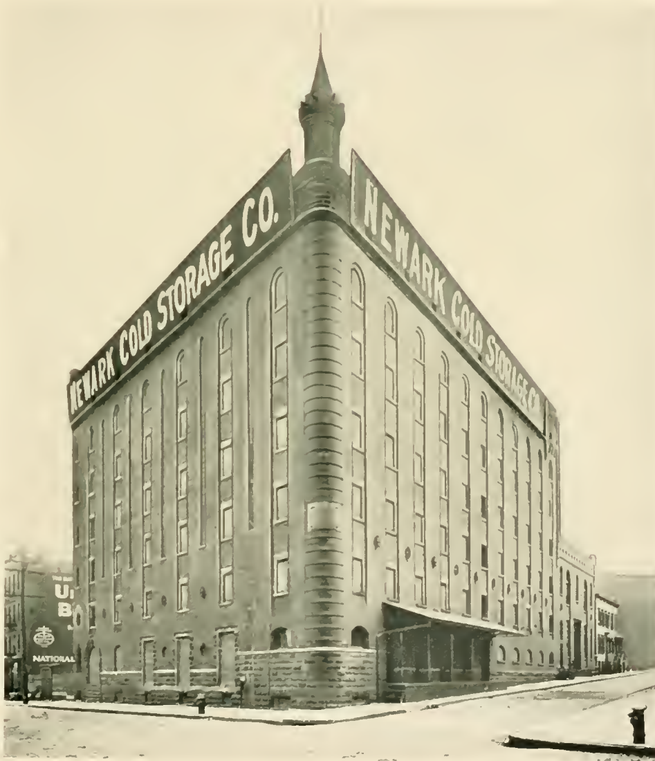
NEWARK COLD STORAGE CO., RIVER AND CHERRY STREETS.
